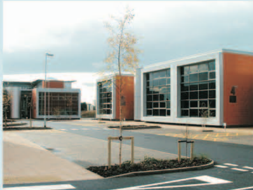
Morton Palms Phase 2 Office Development, Darlington. Design and Build of 13 two-storey office blocks and a three-storey office.
